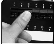
Install color-coded icons (as shown above) or hinged doors provided with modules into area above MAX modules to secure modules into panel. See MAX module instructions for additional details.
